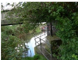
Under the railway bridge (approx. 1.17 miles in)
