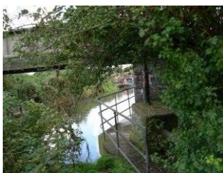
Under the railway bridge (approx. 1.17 miles in)
